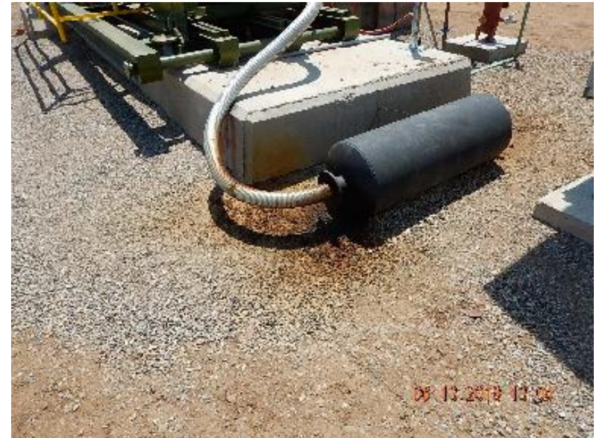
Photo 2: Impacted soil and gravel at exhaust muffler.
