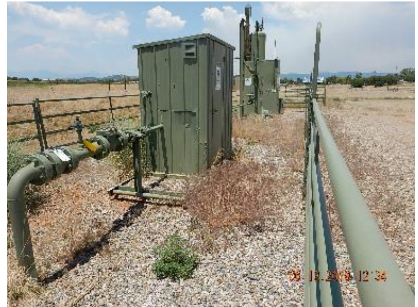
Photo 2: Vegetation inside equipment fencing..
