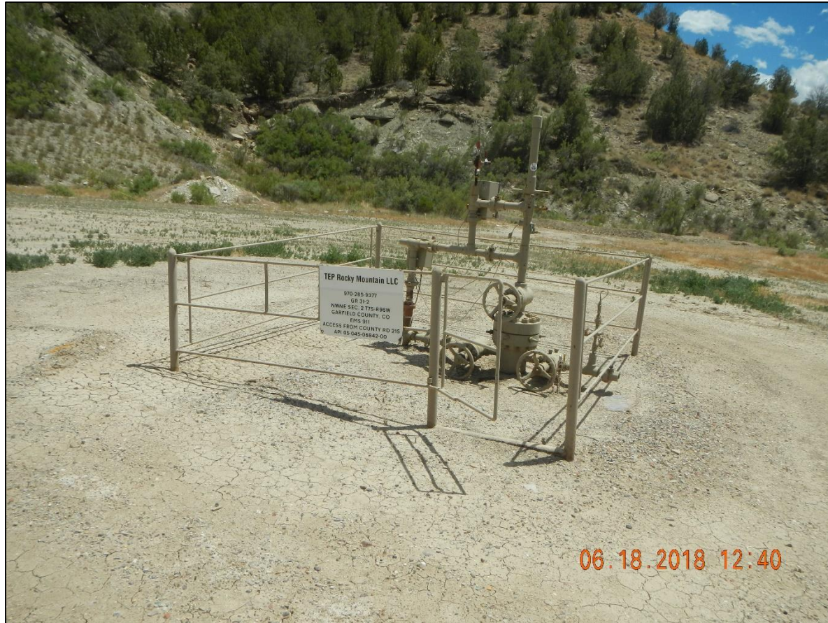
Well head and sign. Weeds coming up around well head.
