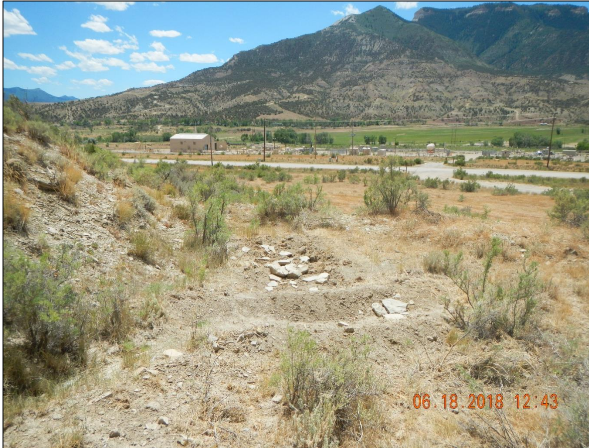
Storm water BMP's have been maintained. Channeling has been repaired.
