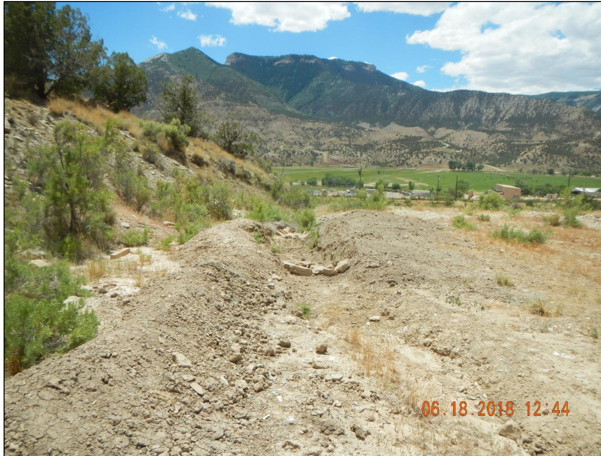
Tubing has been removed. Storm water BMP's have been maintained.
