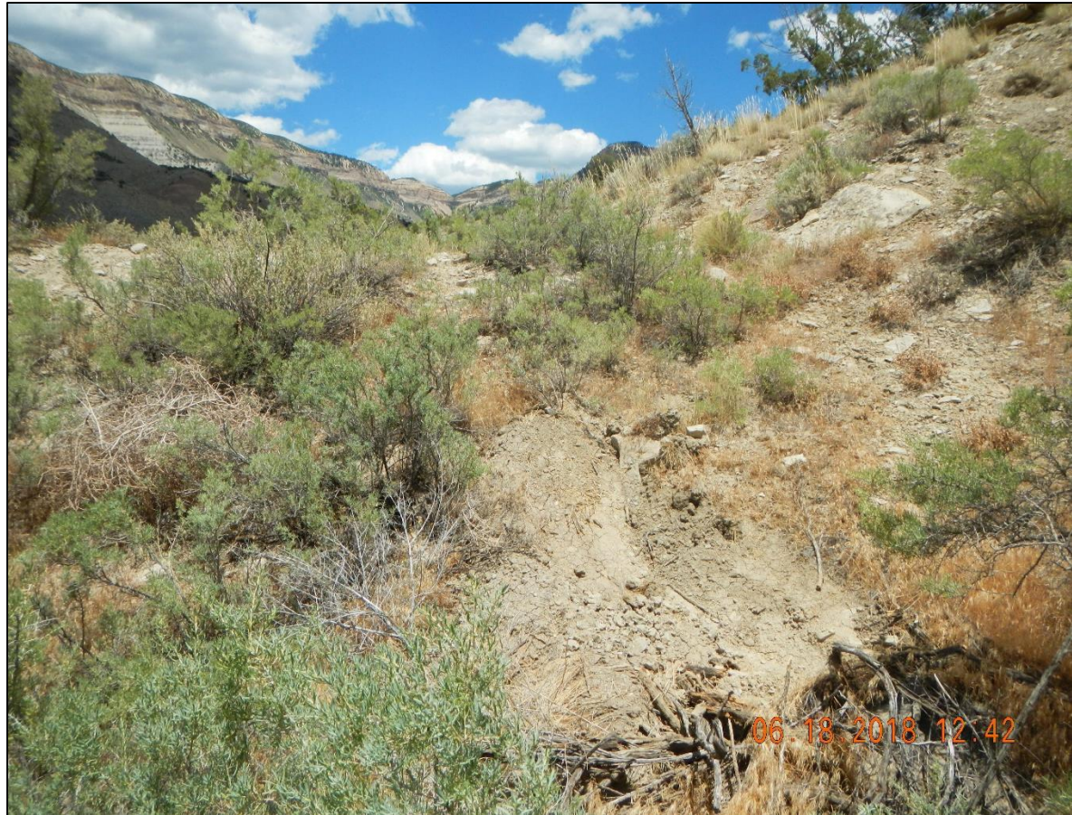
Channeling has been repaired.
