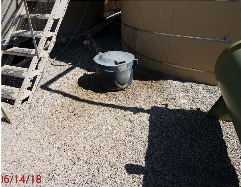
Location Photo #7, Stained rock in containment
