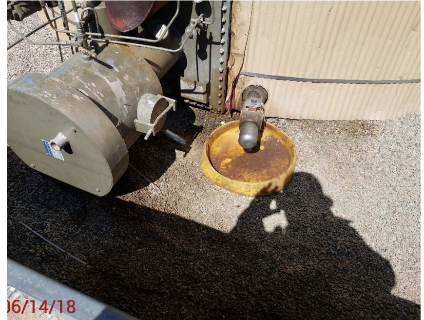
Location Photo #4, Stained rock in containment
