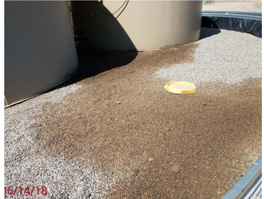
Location Photo #6, Stained rock in containment
