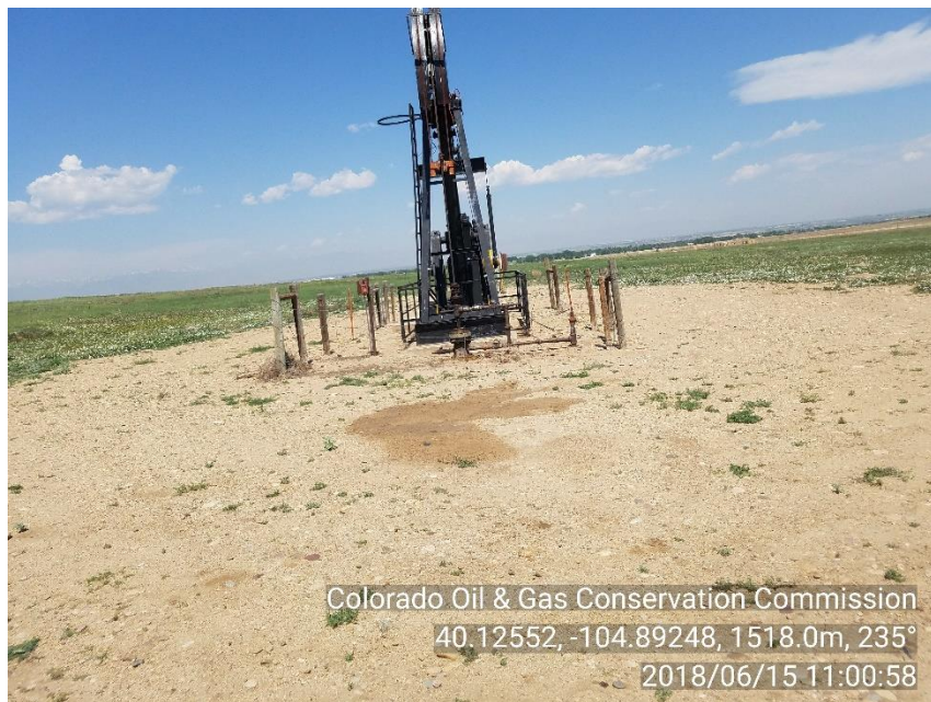
Photo 3. Stained soil east of wellhead
