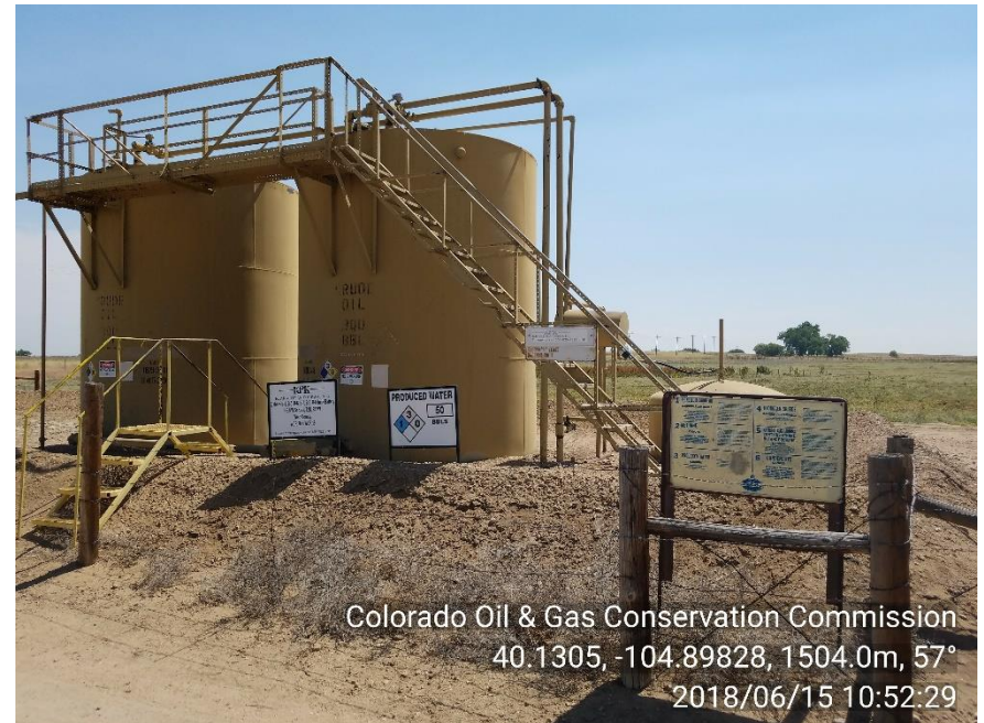
Photo 2. Tank battery
