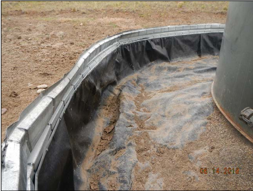
Photo 1. Berm has been repaired.
