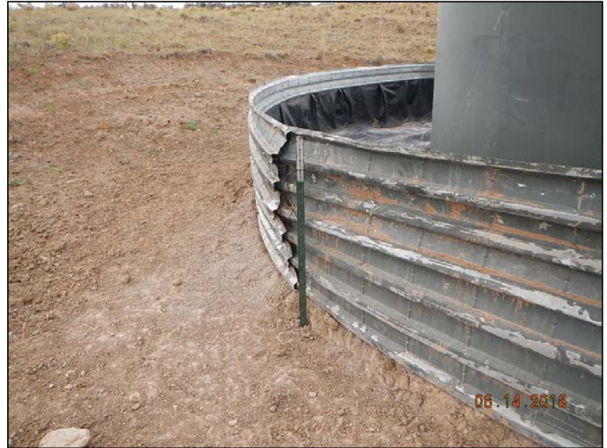
Photo 2. Berm has been repaired.
