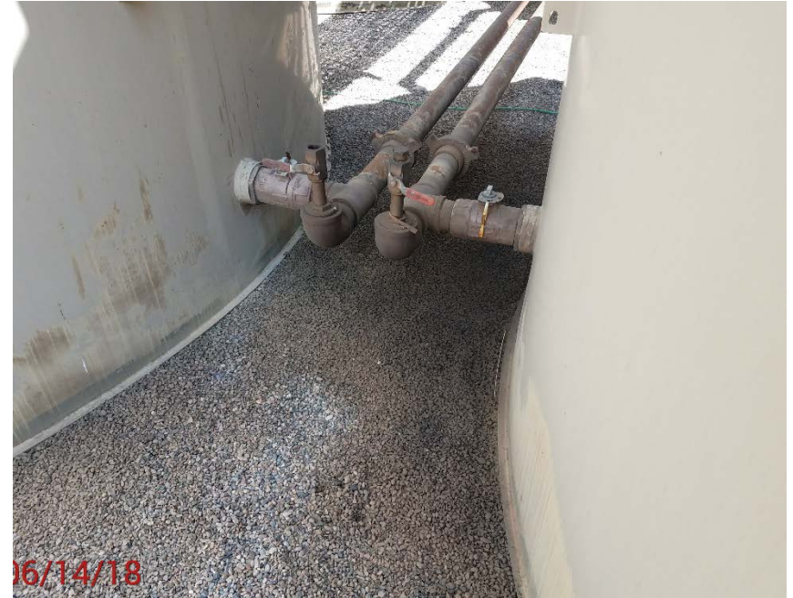
Location Photo #4, Stained rock in tank battery containment
