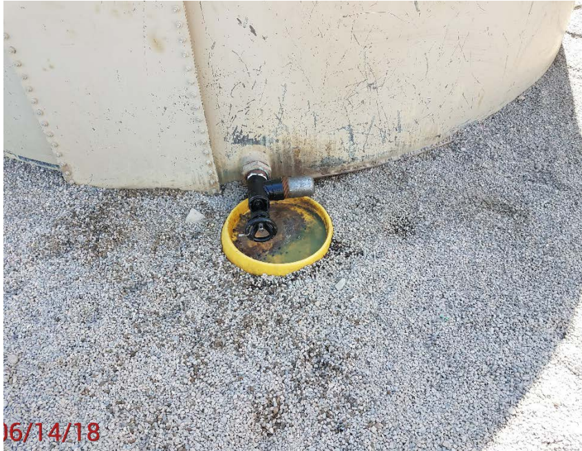
Location Photo #3, Spilled condensate in drip pan
