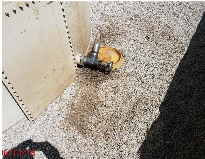
Location Photo #5, Stained rock in tank battery containment
