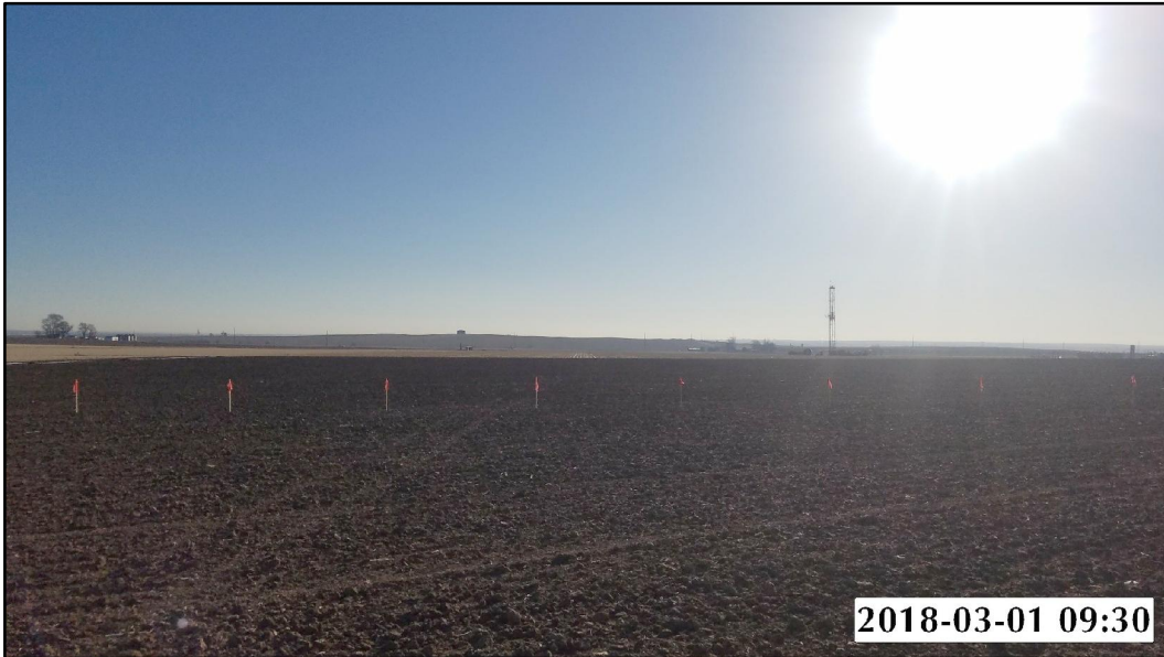
LOCATION PICTURE OF WALTERS 14-21HZ WELL PAD - CAMERA ANGLE EAST
