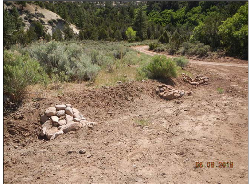
Photo 4. Stormwater BMPs repaired.
