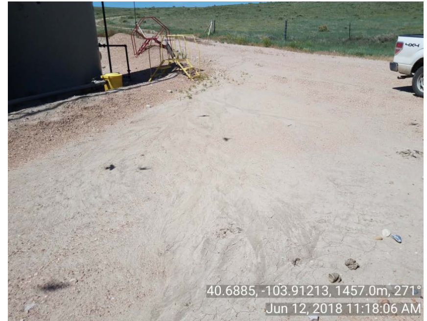
Photo 5: Stormwater erosion on NW side of location
