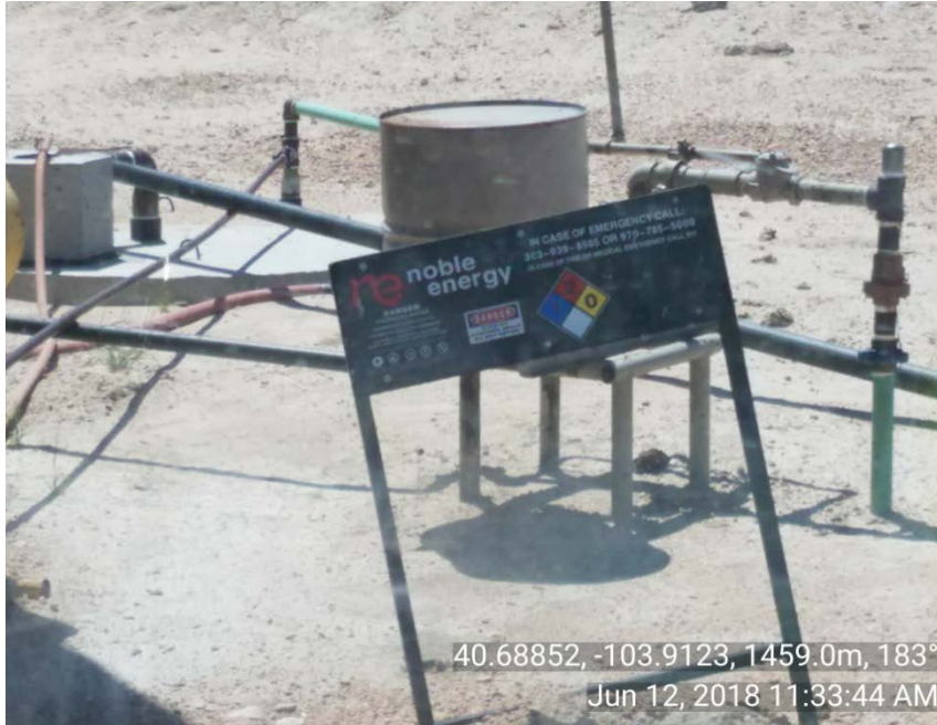
Photo 6: No capacity on water vault sign
