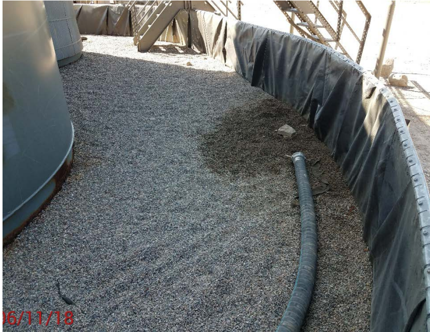
Location Photo #1, stained rock in tank battery containment.
