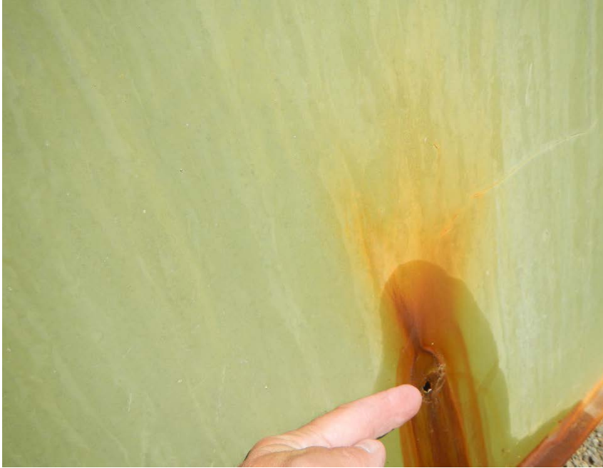
Corrosion hole in 300 bbl PW AST
