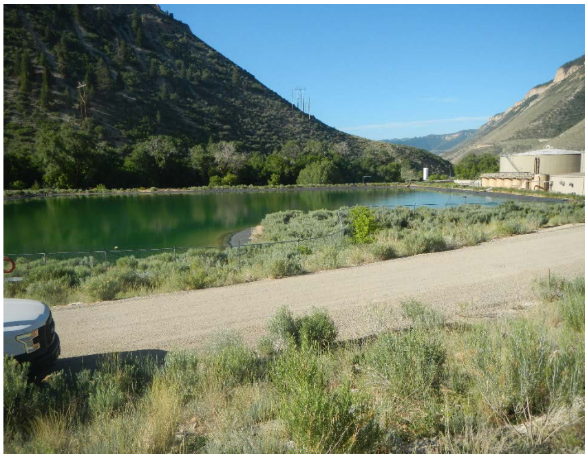
Pit and ASTs looking Southwest
