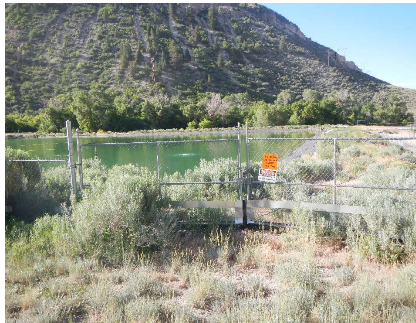
West berm of pit showing weed growth and aerator looking south
