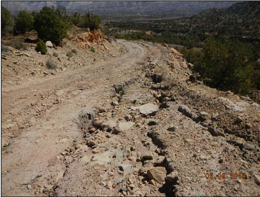
Photo 3. Erosion and sediment migration along access road.
