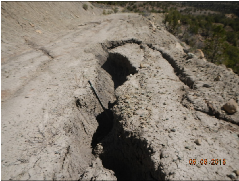
Photo 4. Erosion and sediment migration along access road. Up to 3 feet deep. (See stake in center of photo)
