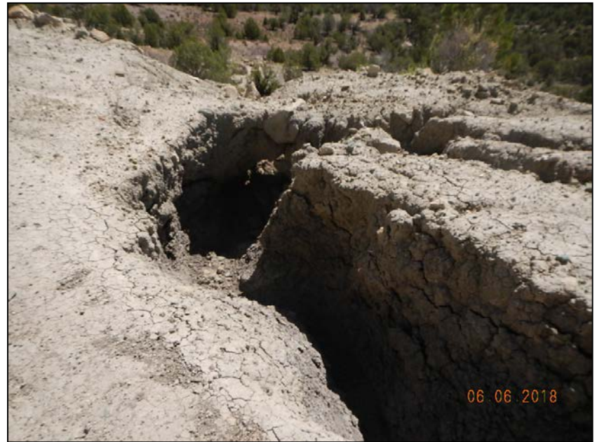
Photo 5. Erosion and sediment migration along access road.
