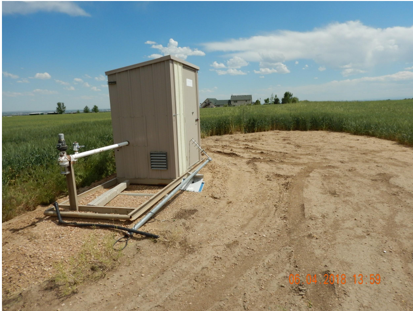
Photo 1. Photo taken from the battery location, facing South. A gas meter run has been left on location. Operator should have removed the equipment per Rule 1004 by 4/4/2017.
