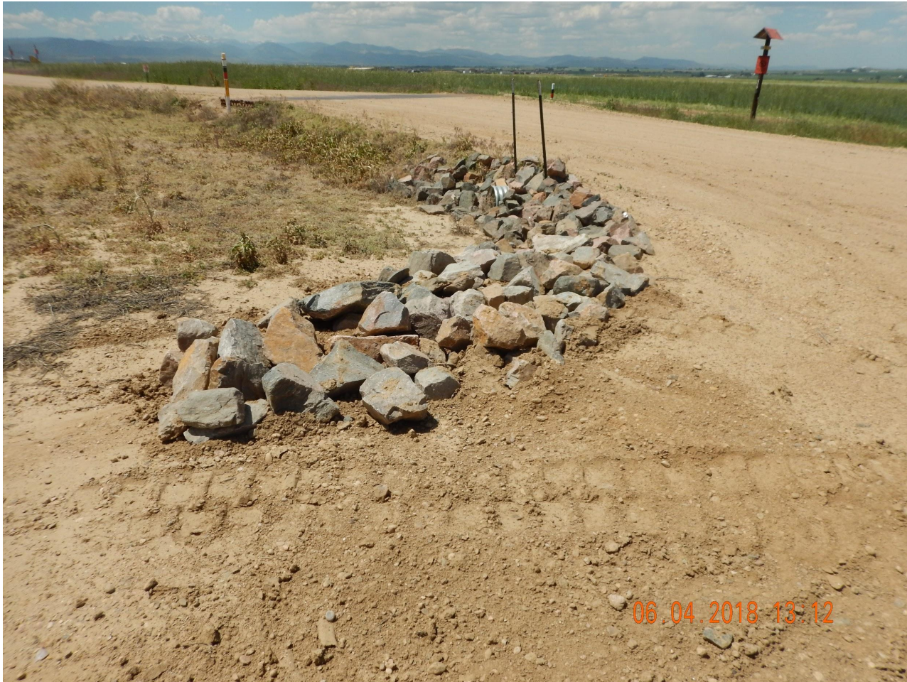
Photo 3. Photo taken from the entrance of the battery location, facing West. Operator has installed rip-rap and armored around the culvert.
