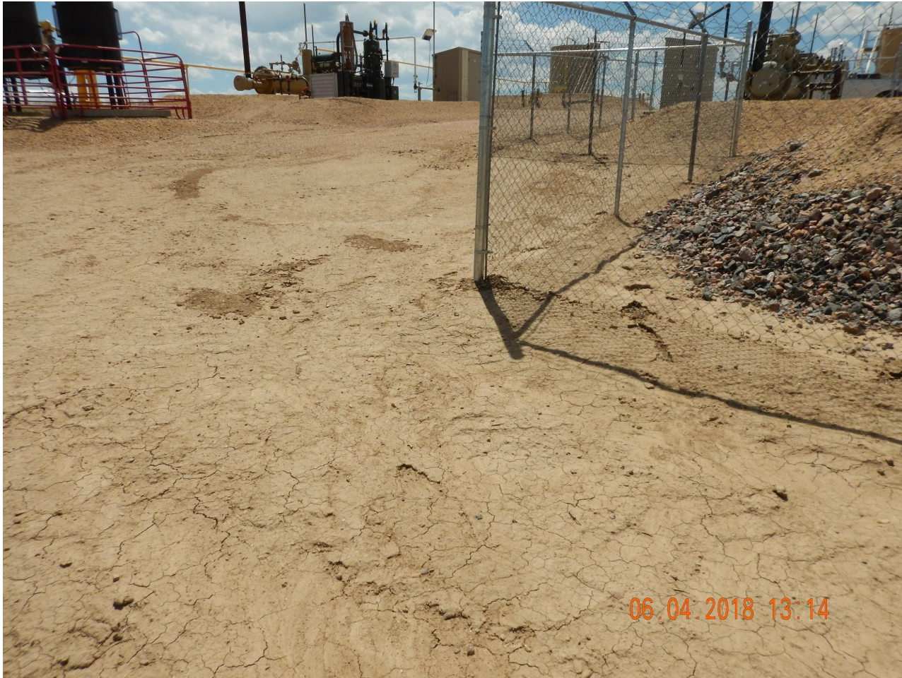
Photo 2. Photo taken from the eastern battery location, facing West. Operator has made repairs to the rill erosion.
