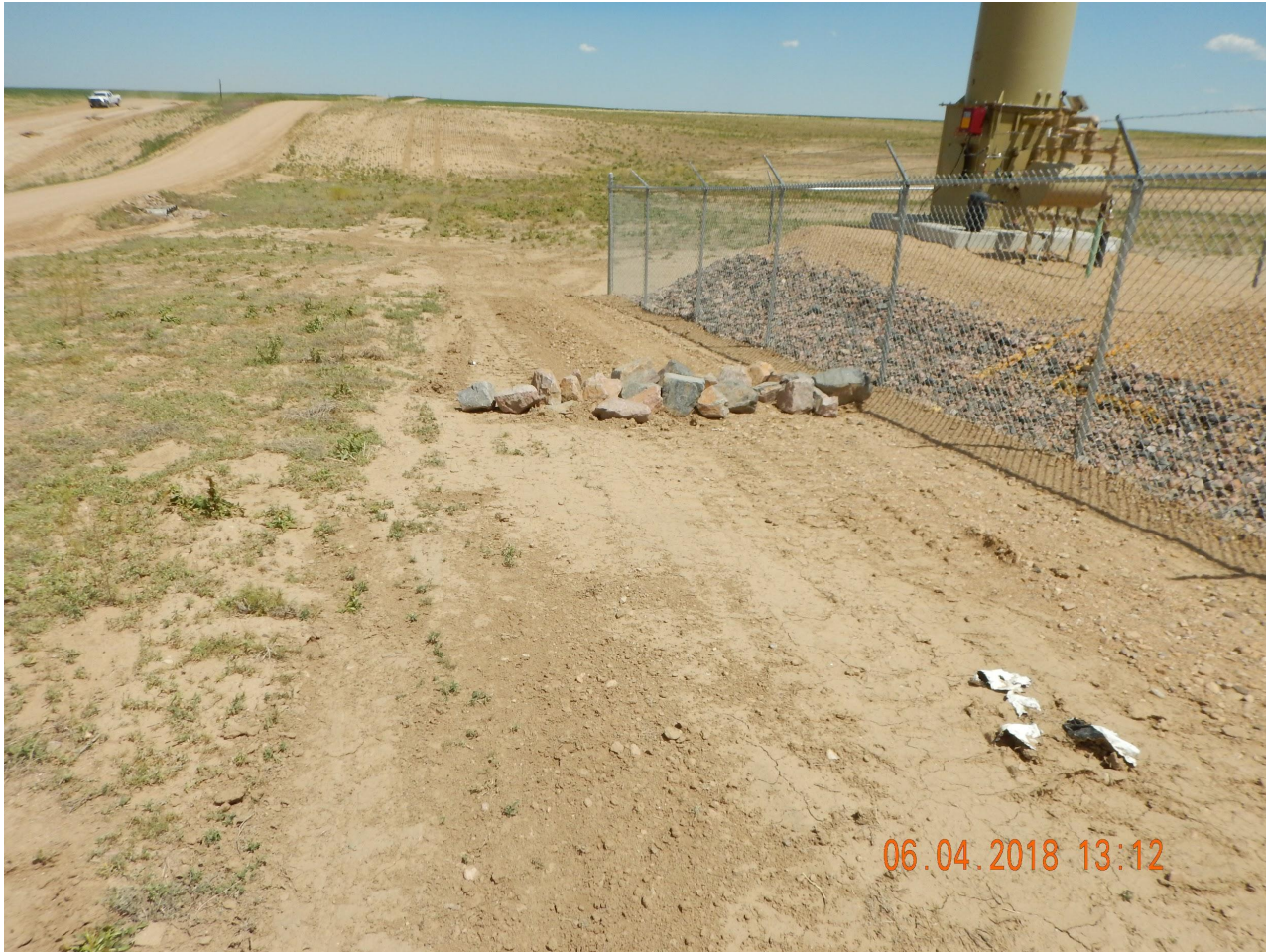
Photo 1. Photo taken of the northern battery location, facing East. Operator has made repairs and installed a check dam.
