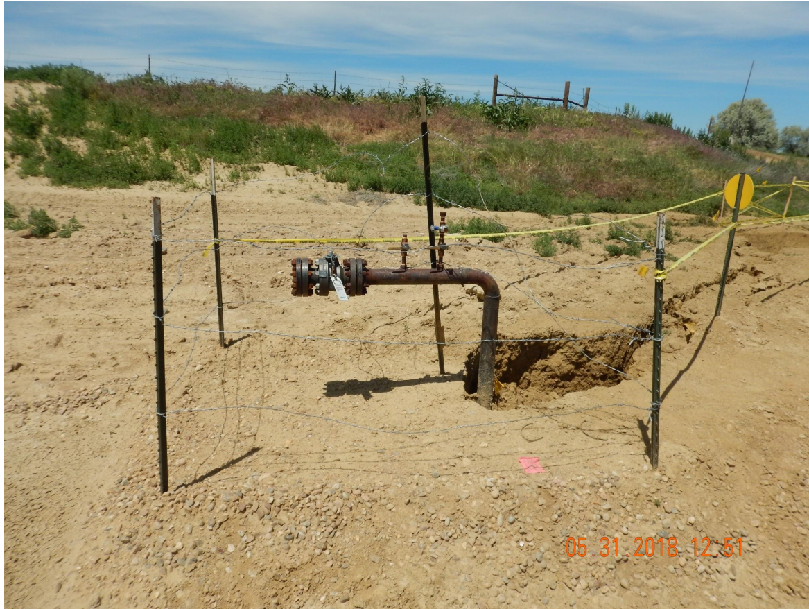
Photo 1. Photo taken from the battery location, facing North. Riser remains at the battery location and should have been removed by 11/31/2017.
