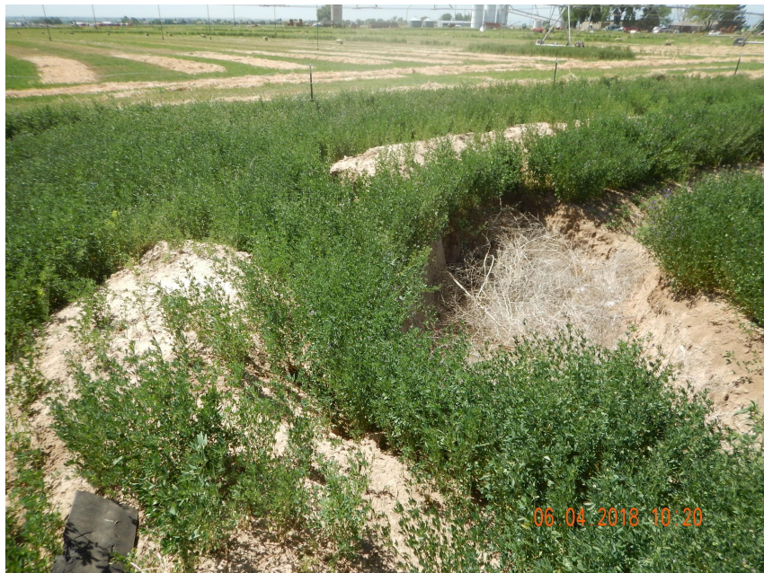
Photo 5. Photo taken from the southeast perimeter of location, facing South. Photo illustrates the southeastern sediment trap. Weed debris was observed inside the sediment trap.
