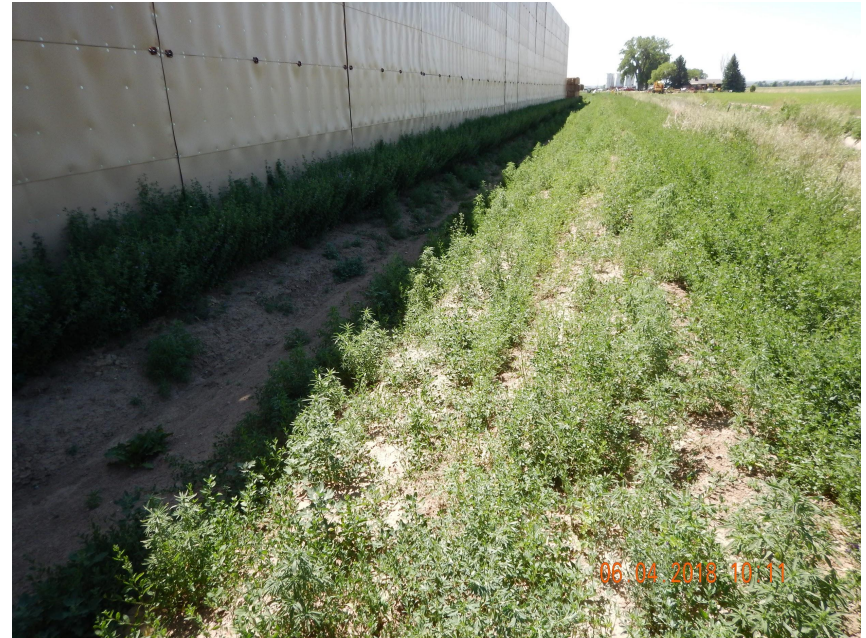
Photo 2. Photo taken from the northwest perimeter of location, facing South. Ditch and berm BMP has been installed around the entire perimeter of the location. Alfalfa has established throughout the stormwater area, including the berm BMP, but other undesirables like Kochia and Canada thistle were also observed. Operator shall control all noxious and undesirable weed species on cropland.
