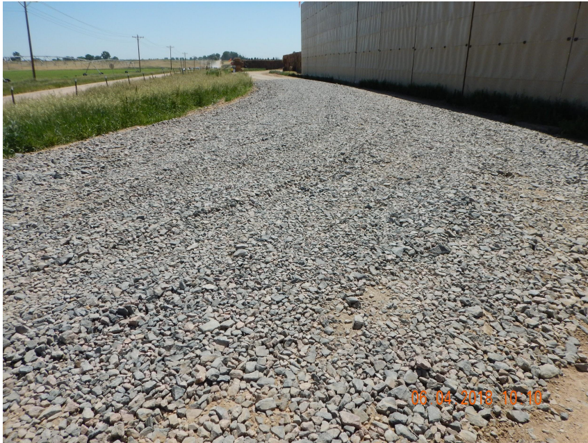
Photo 1. Photo taken from the entrance of location, facing East. Vehicle tracking device has been installed and appears to be in proper functioning condition.
