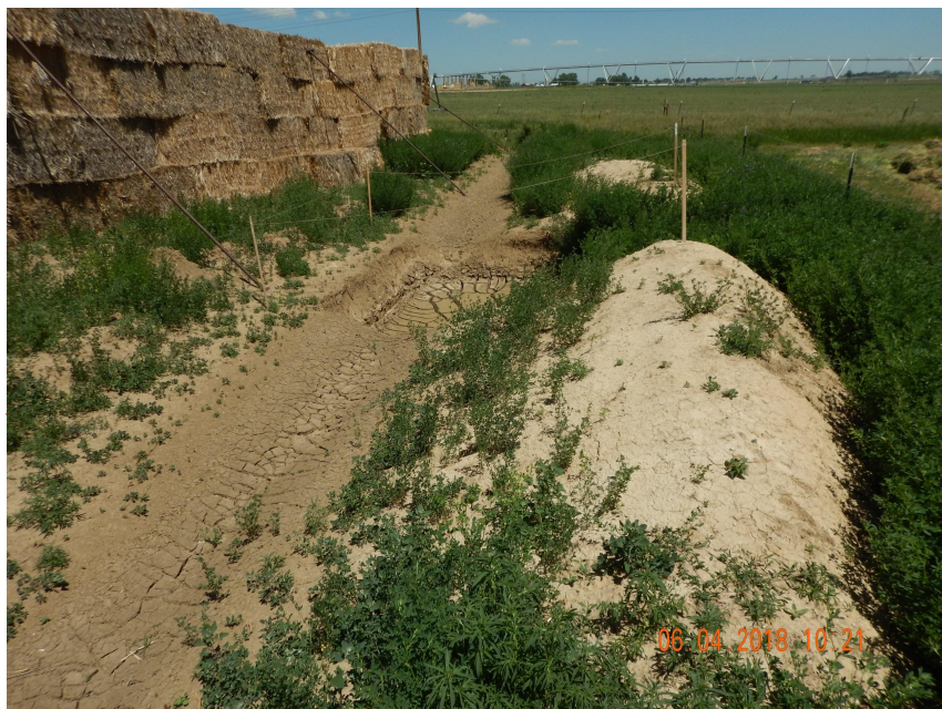
Photo 7. Photo taken from the northeast perimeter of location, facing North. Photo illustrates the northeastern sediment trap that appears to be properly functioning.
