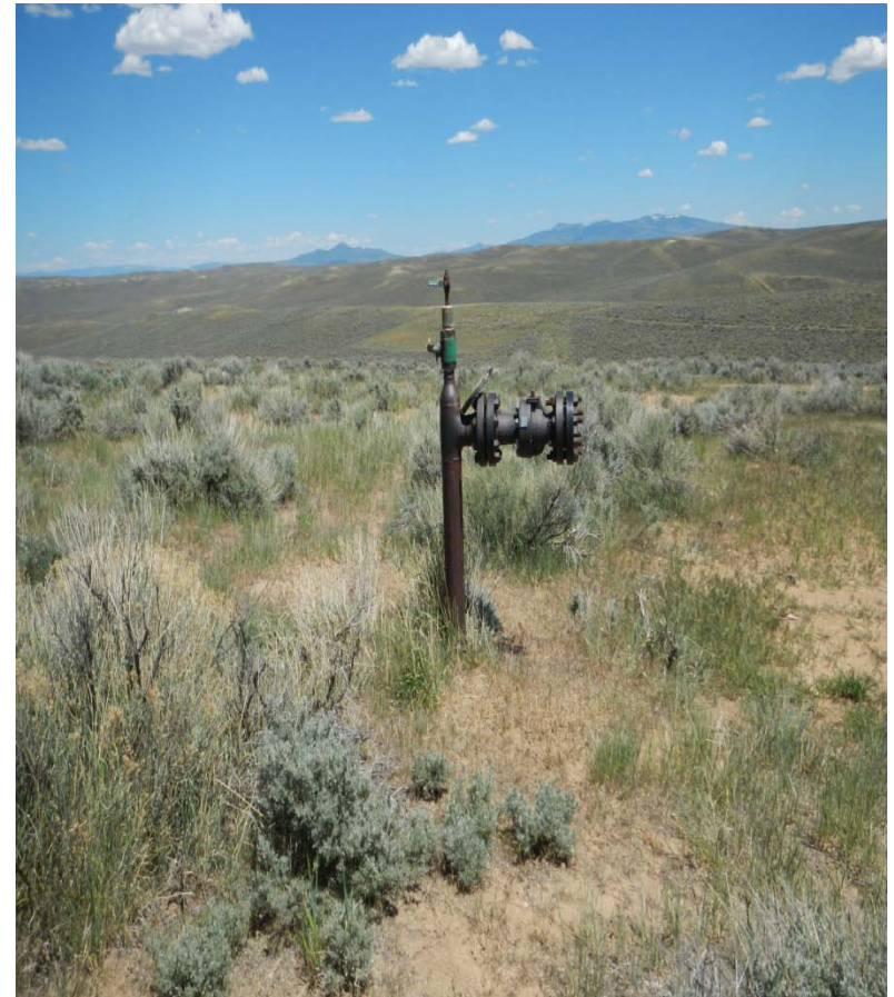
Photo#6: Pipeline Riser (?) in area where Access Road meets main road.
