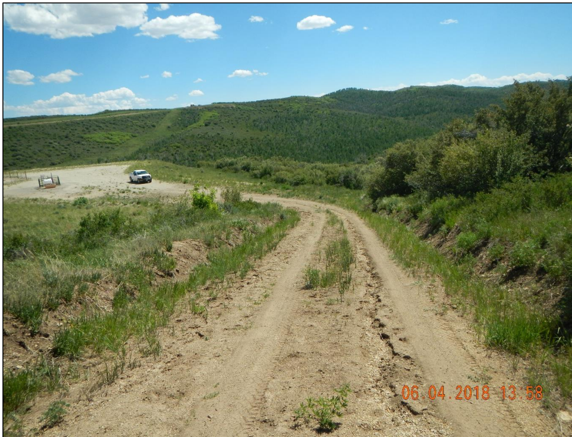
Washing and riling of rut on road.
