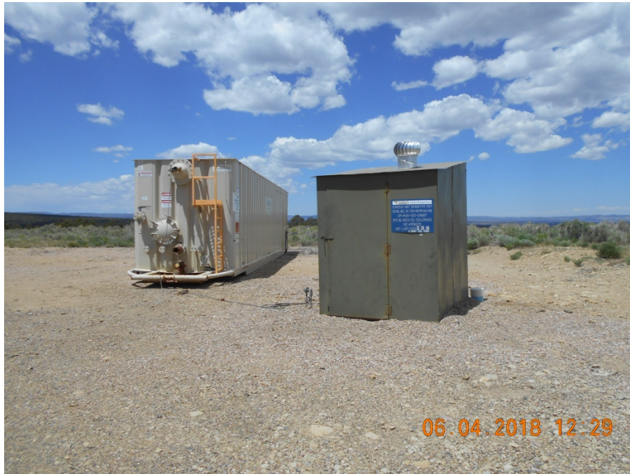
Injection wellhead inside housing
