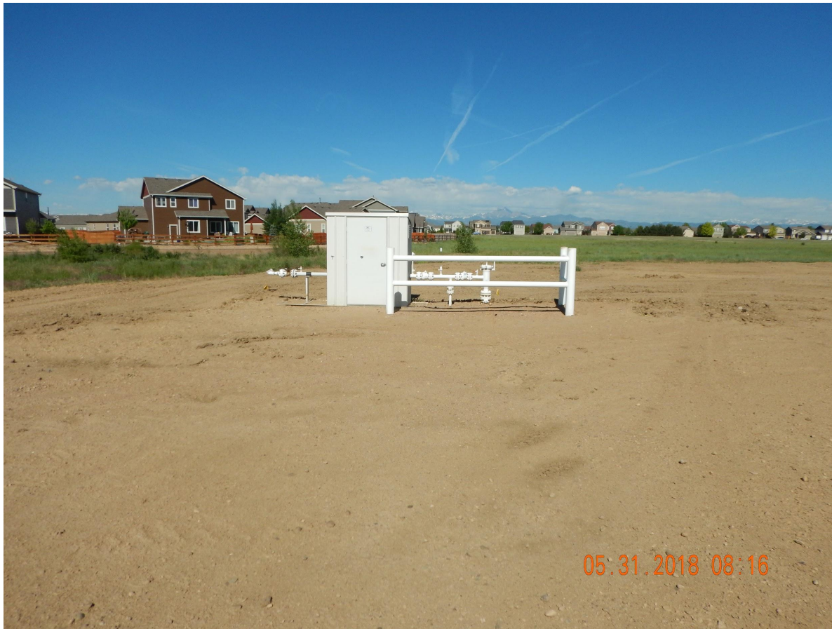
Photo 3. Photo taken from the southern facility/well location, facing West. Operator shall remove the remaining equipment per Rule 1004 by 7/25/2018.
