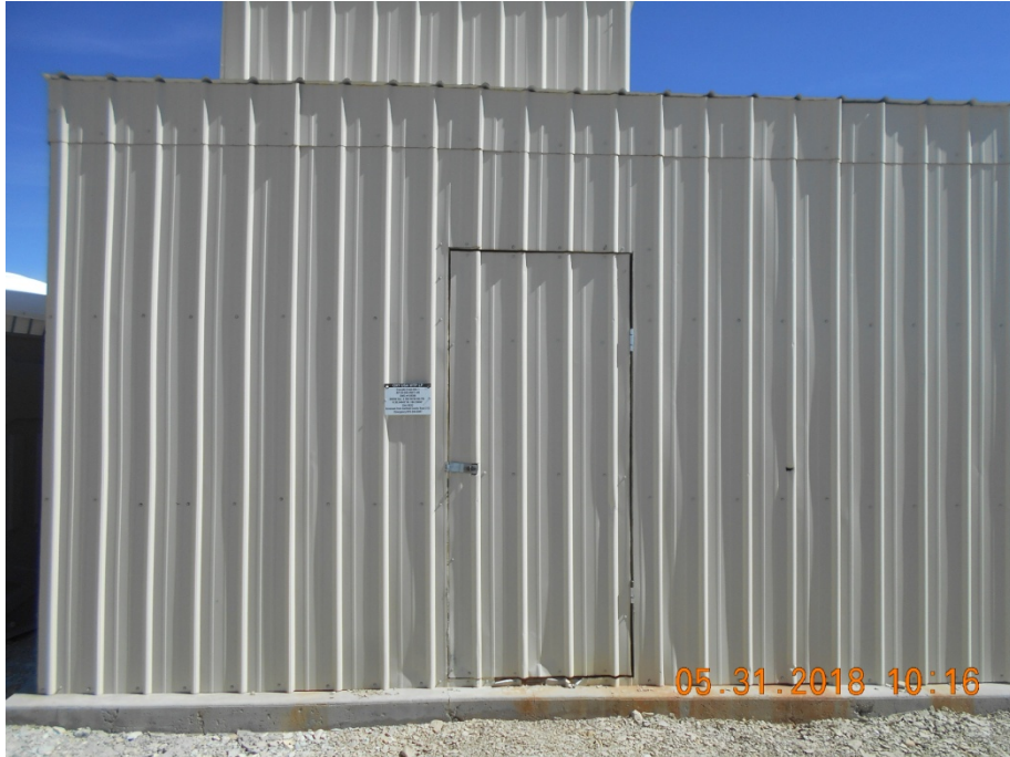
Injection wellhead housing with sign
