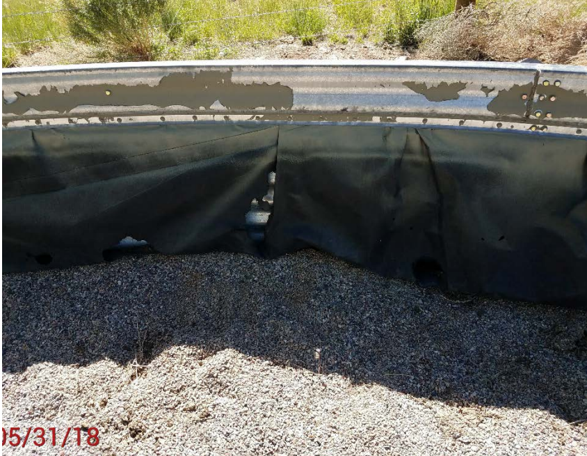
Location Photo #5, holes in battery liner
