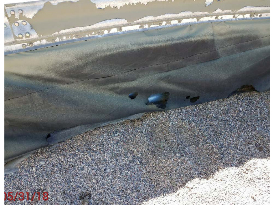
Location Photo #4, holes in battery liner
