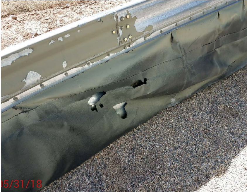
Location Photo #3, holes in battery liner
