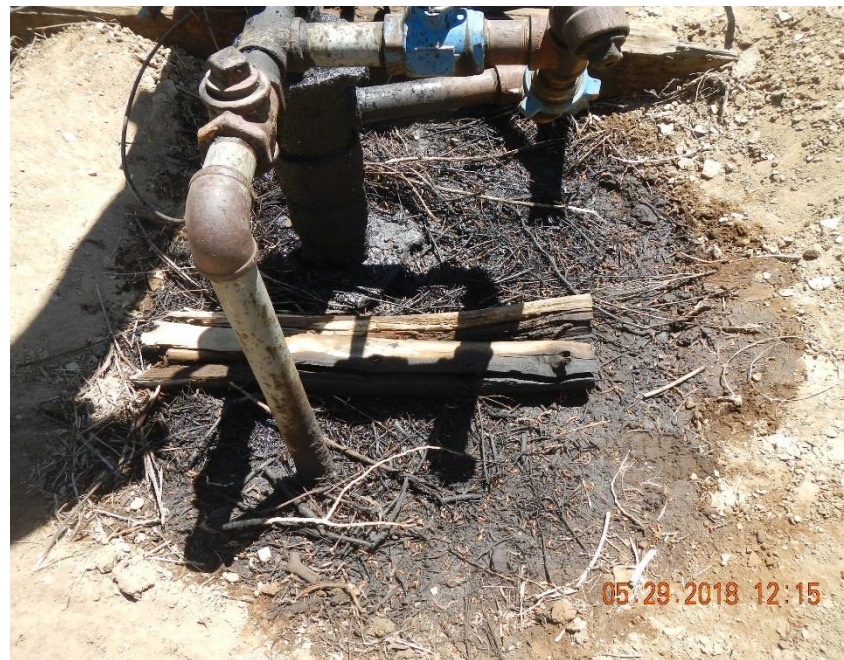
Well head is wet and surrounded by stained soil.
