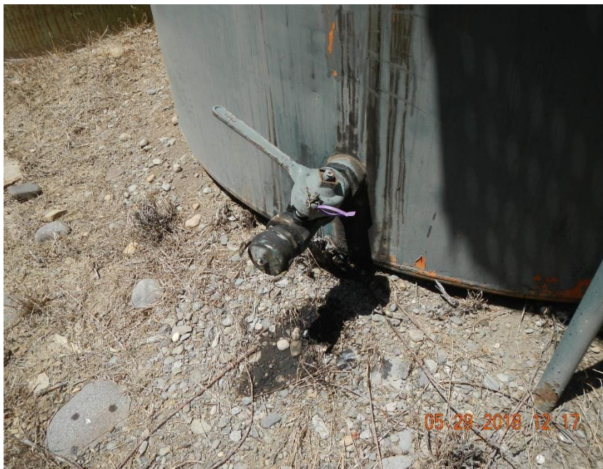
Stained soil beneath load out valve on AST. Tank is stained with oil, noted on previous inspection.
