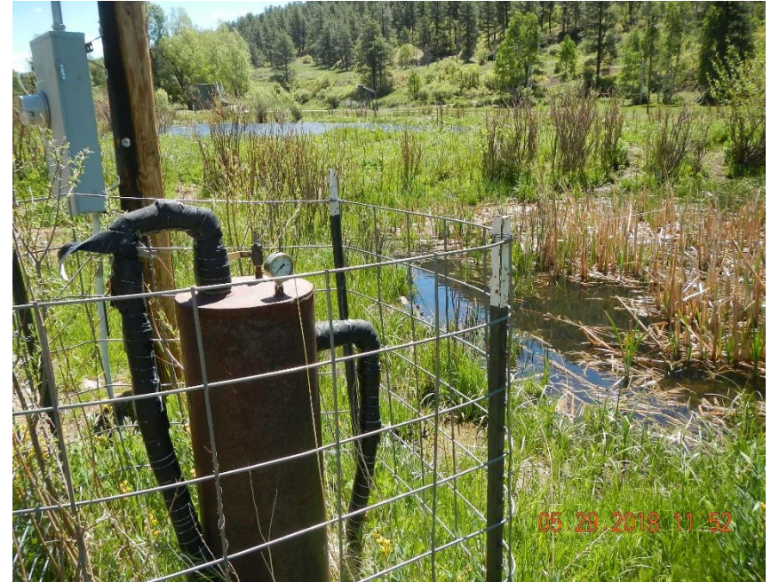
Drop out tank with 4 psi on pressure gauge.
