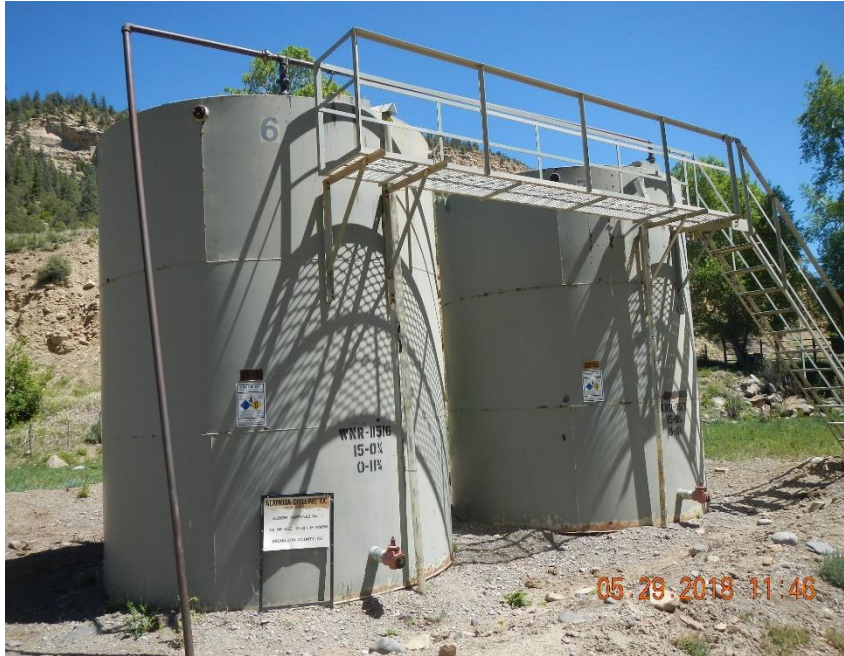
Albert Martinez #1 tank battery. Secondary containment berm shared with Nielson #4.
