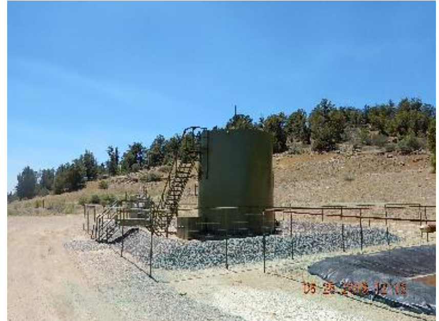
Photo 4: Approach side of tank and NFPA labels are not visible.
