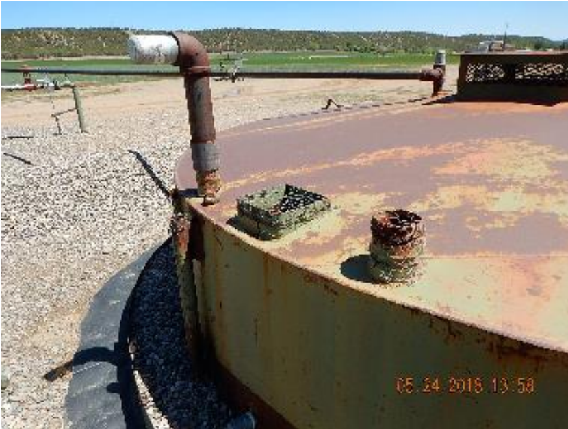
Photo 3: Covered tank opening.
