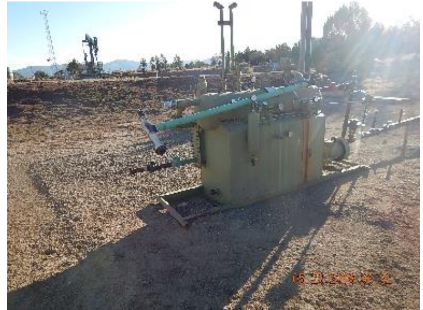
Photo 2: Separator with disconnected flow line.
