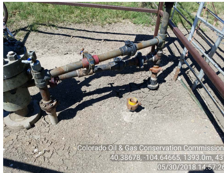
Wellhead detail; Corrective Action: Flowline risers not LO/TO or marked are considered unused equipment
