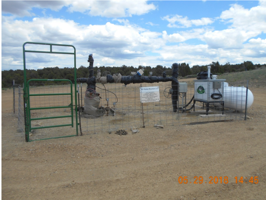
Injection wellhead with sign.
