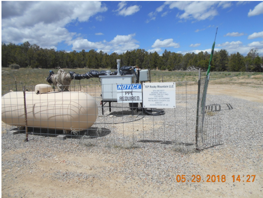
Injection wellhead with sign.
