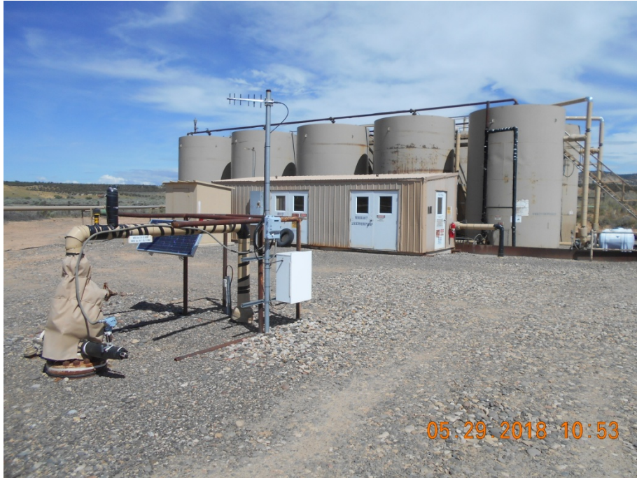
Injection wellhead, pump housing and tank battery
