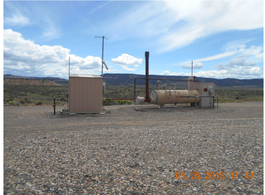
Meter housing and Separator
