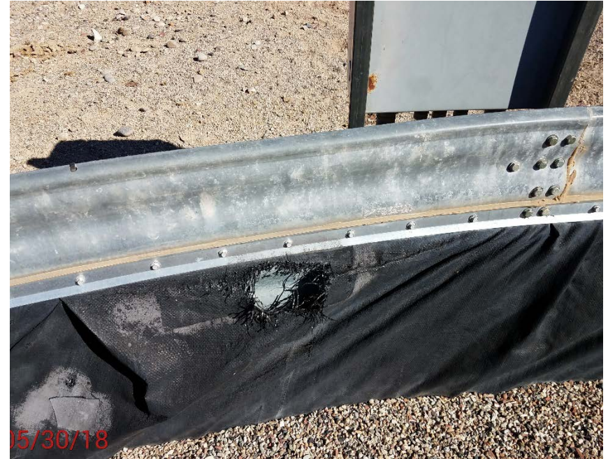
Location Photo #4 holes in containment liner
