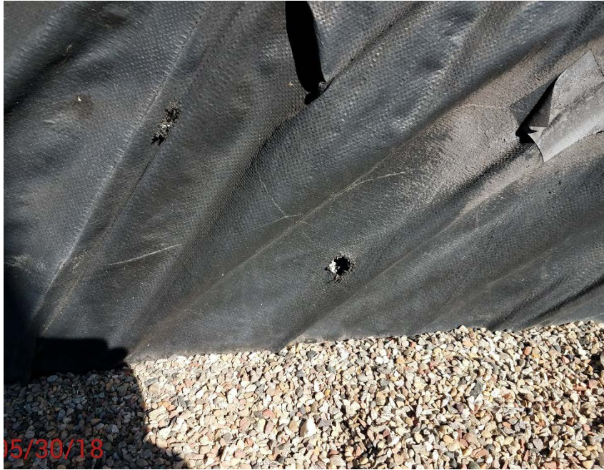
Location Photo #5 holes in containment liner
