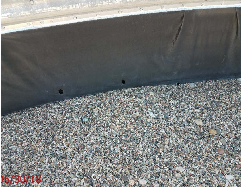
Location Photo #3, holes in containment liner
