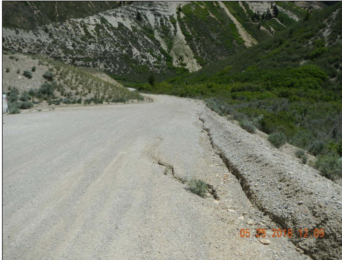
Erosion rill on lease road.
