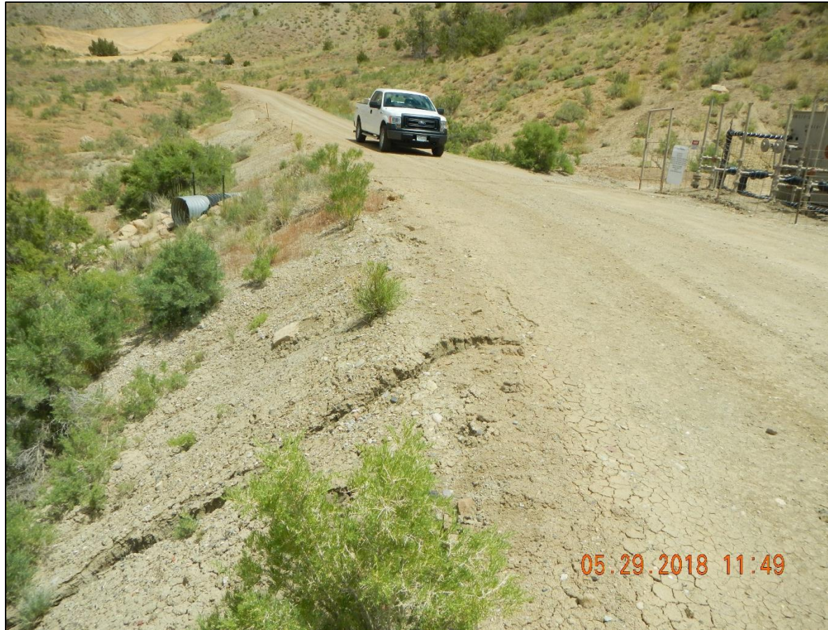
Erosion of roadside of road across from the separators.
