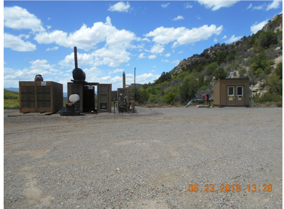
Pump housing, Separator and Generator
