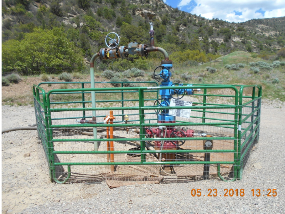
Injection wellhead with fencing
