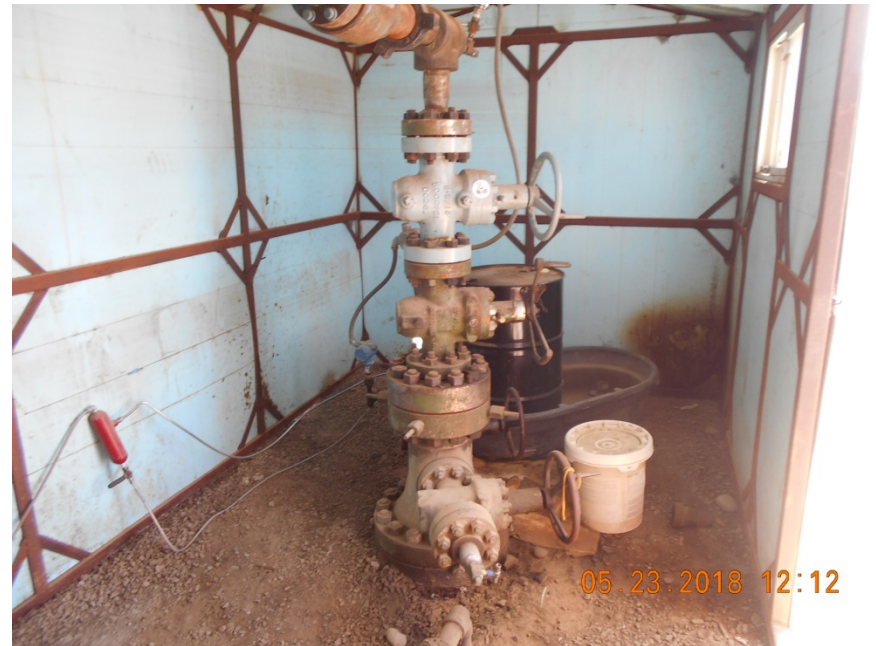
Injection wellhead inside housing
