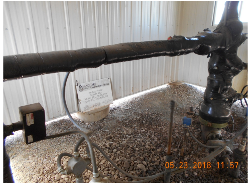
Injection wellhead inside housing
