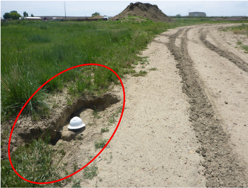
Photo 7. Photo taken from the South end of the access road between the well and the facility, facing West. Appears stormwater runoff is causing rill erosion along the remaining access road between the well and the facility.
