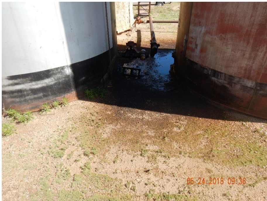
Photo 7: Photo taken from the south end of the tank battery. Photo shows what appears to be crude oil is leaking from the southwestern tank.
