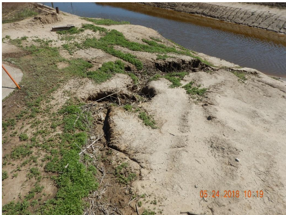
Photo 31: Photo taken from the western edge of the central pit. Photo show gully formation due to stormwater erosion.
