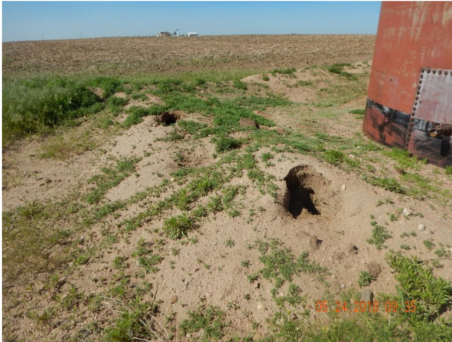
Photo 5: Photo taken from the south end of the location, at the tanks, facing southwest. Photo shows undesirable weedy plant establishment on the berms. Photo also shows wildlife appears to have created burrows/holes within the side of the berms.
