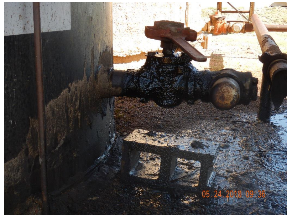
Photo 8: Photo taken from the south end of the tank battery. Photo shows what appears to be crude oil is leaking from the valve of the southwestern tank.
