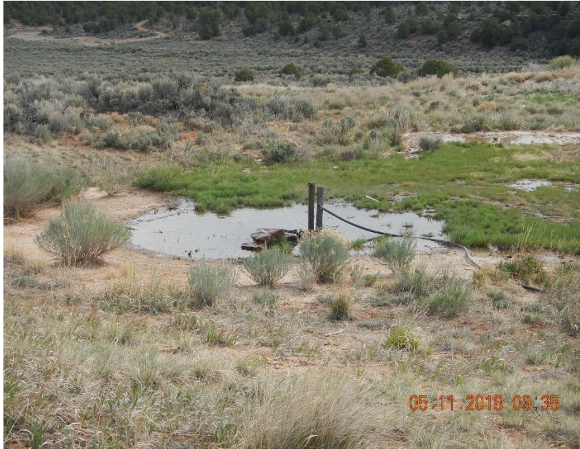
Cathodic protection well located on Meridian Hodges Pool Unit #1 location.
