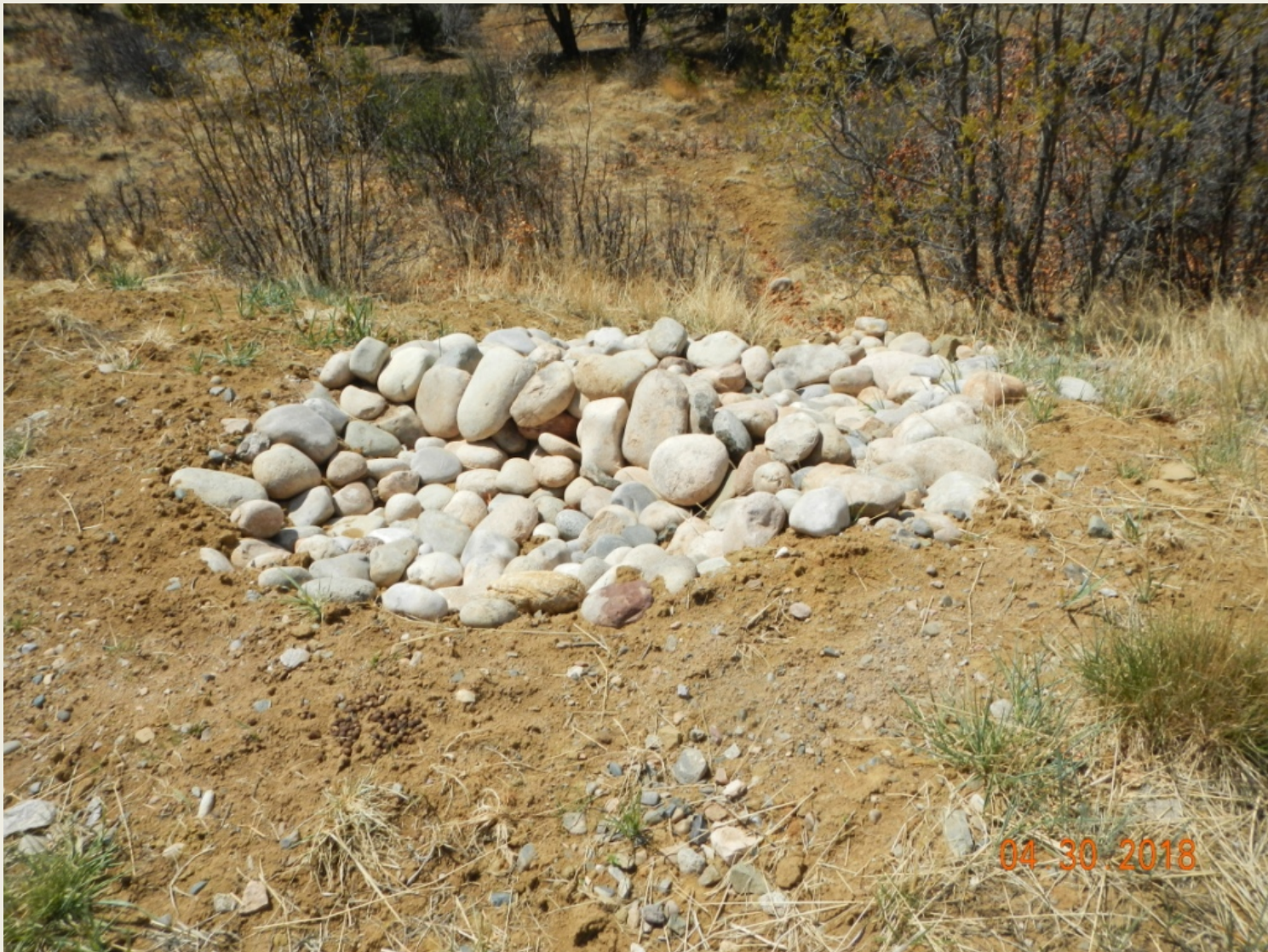
Photo 3. View of a new cobble run-down in the southwestern project area.
