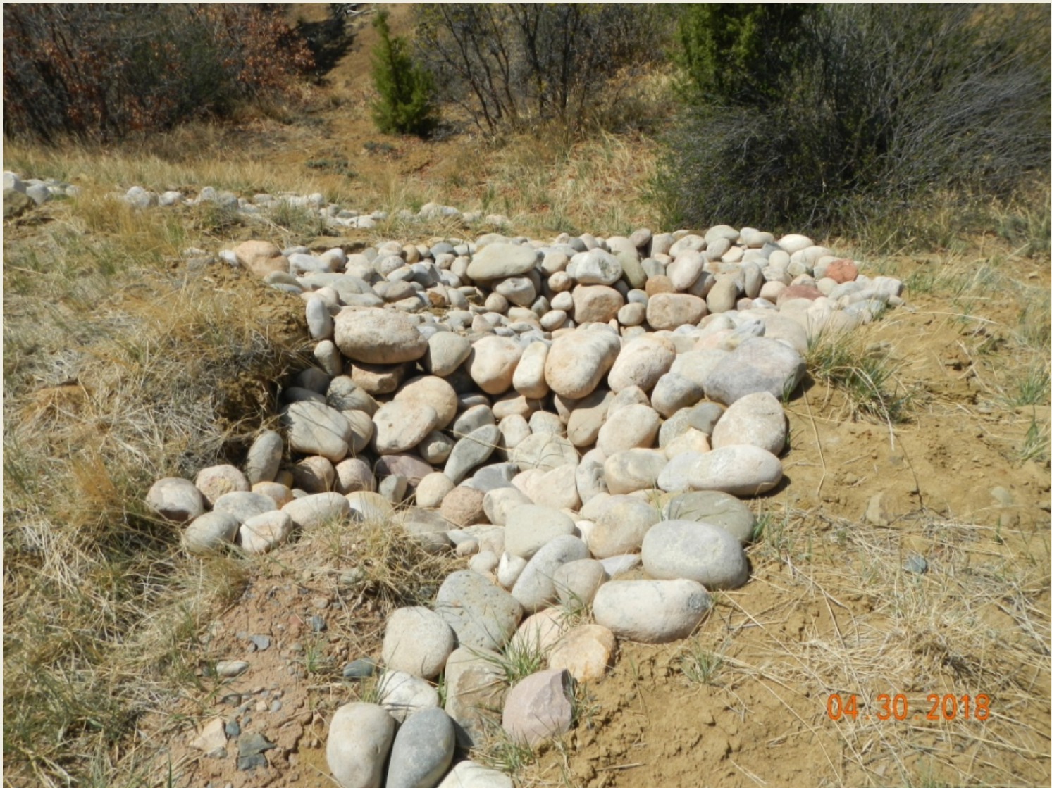
Photo 1. View of cobble run-down in the western portion of the project area.
