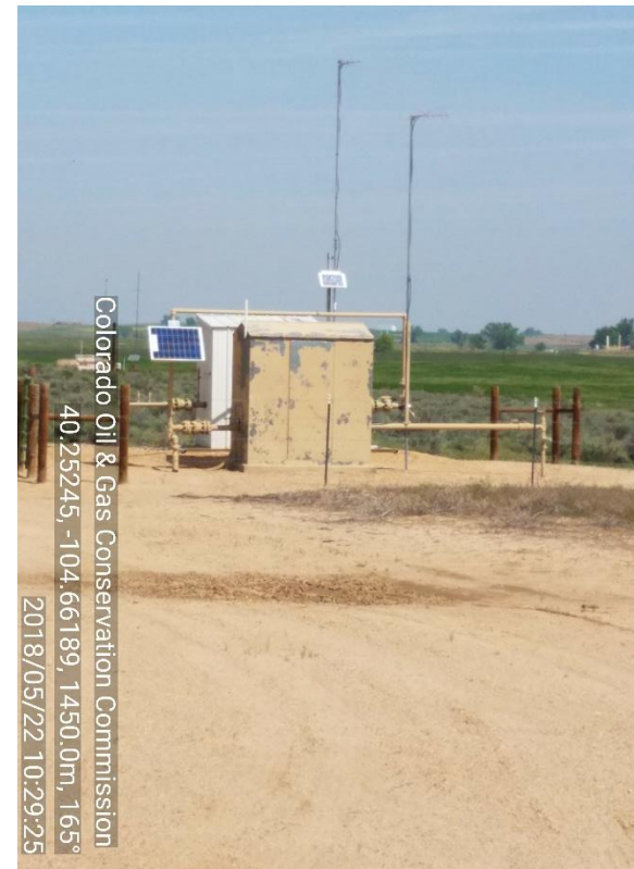
Photo 6 Gas Meter Run
