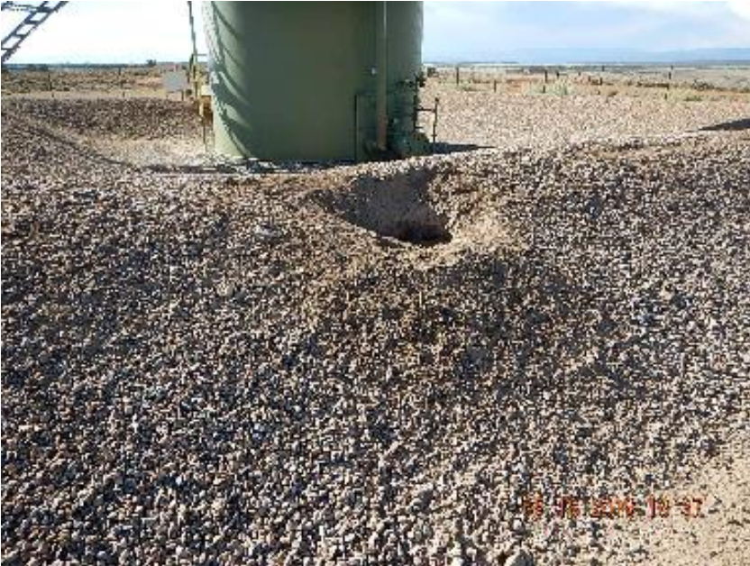
Photo 3: Animal burrow in tank containment berm.
