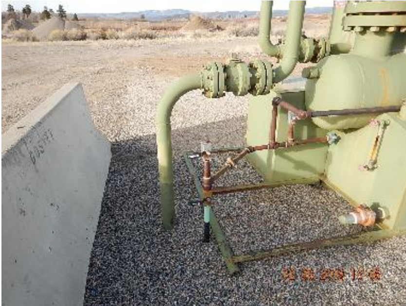
Photo 3: Unused 1" gas line at separator previous inspection.
