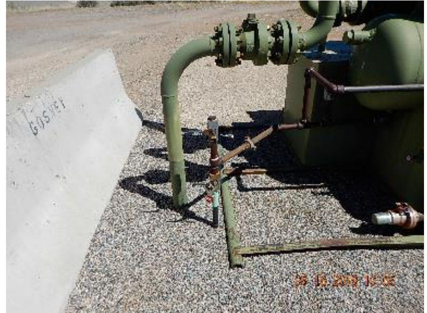
Photo 4: Locked out 1" gas line at separator.
