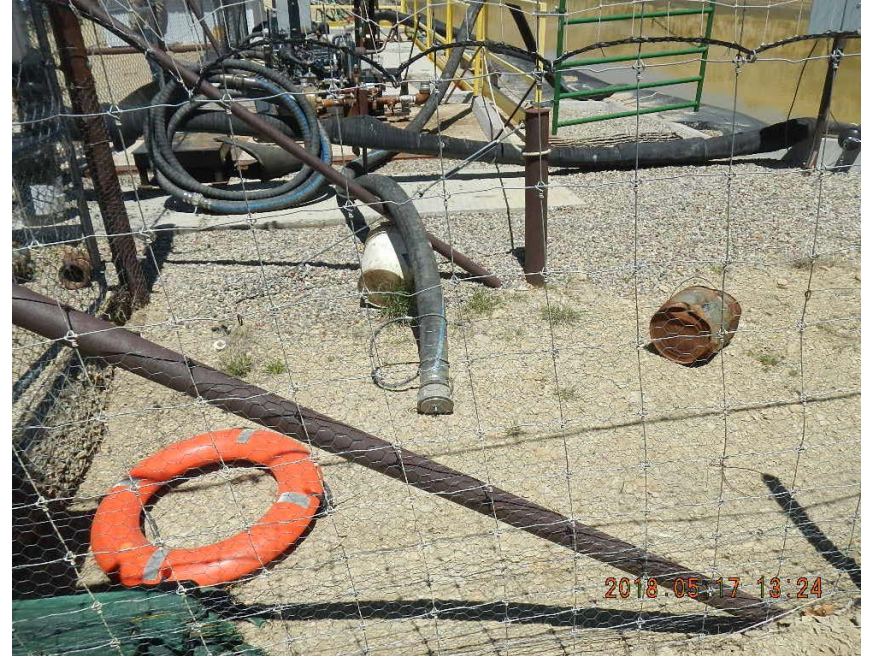
Debris (buckets), hoses on liner
