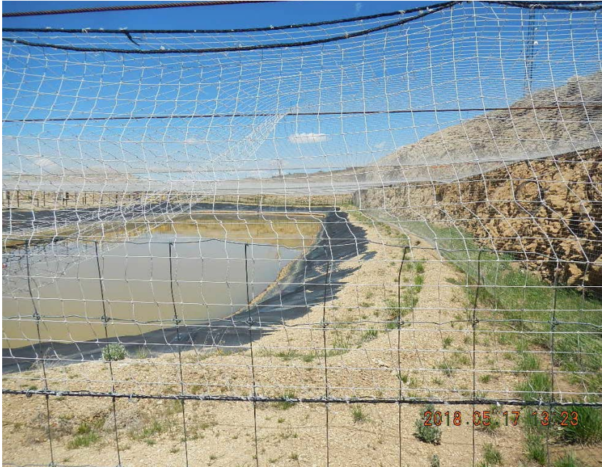
Holes in netting
