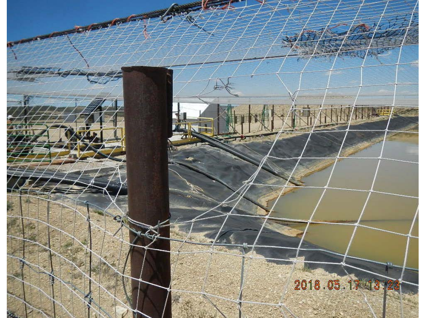
Holes in netting
