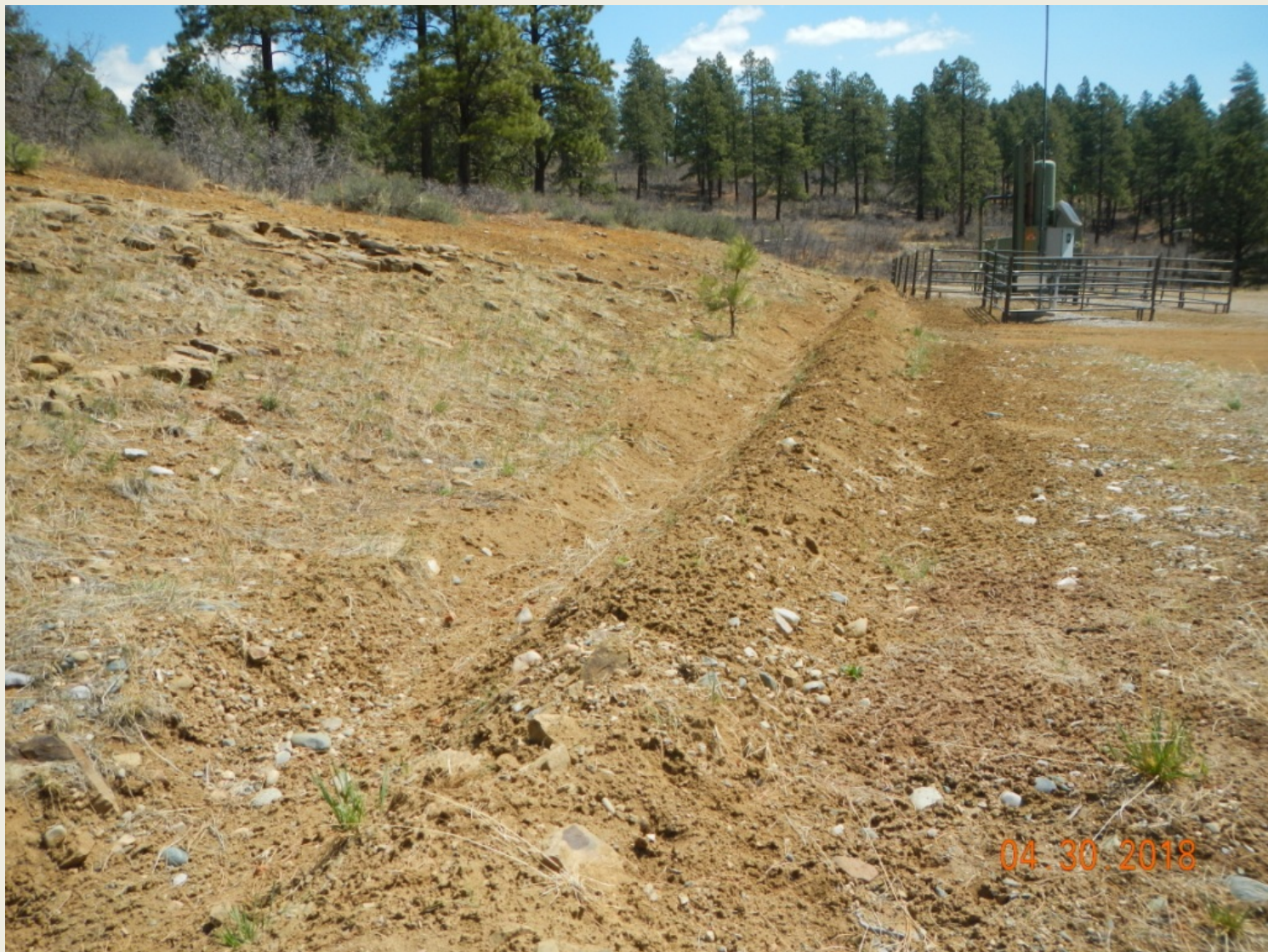
Photo 3. View of recently graded diversion and berm. Seedlings observed on berm.
