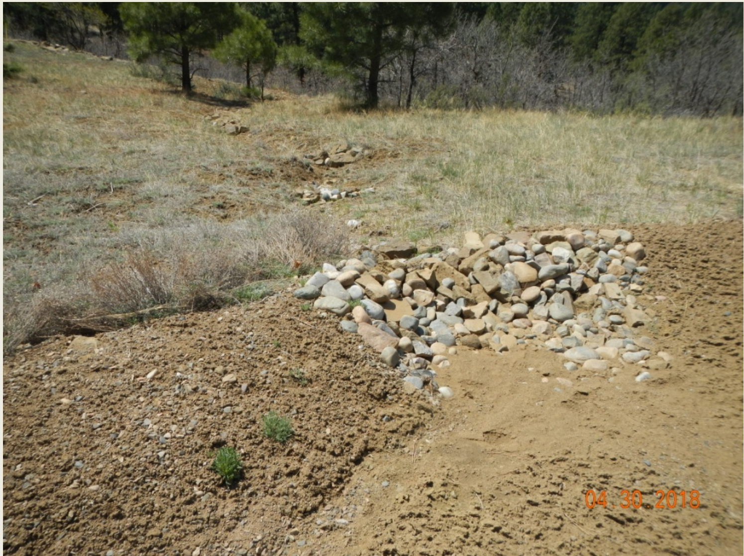
Photo 1. View of check dams in the southern portion of the project area. Appear to be functioning.
