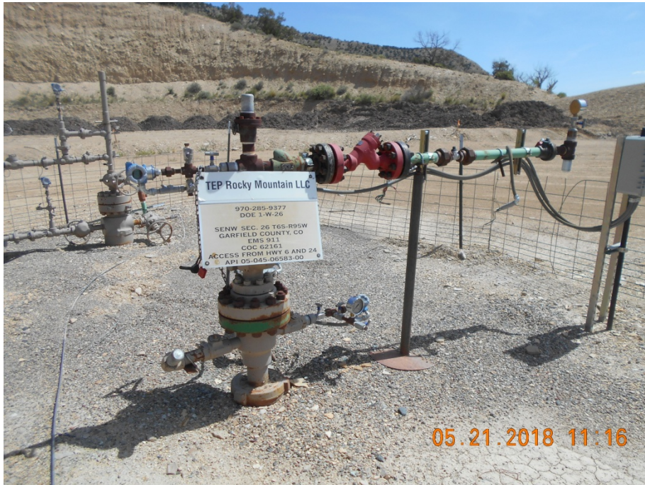
Injection wellhead with sign.
