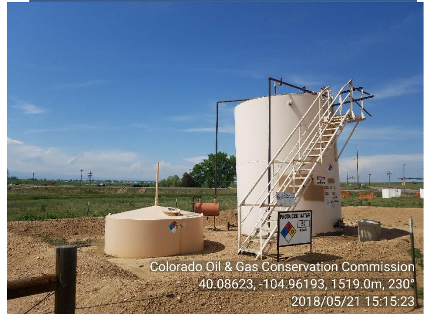
Photo 2. Tank battery
